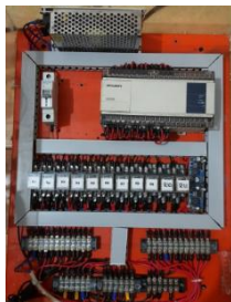
Figure 6. Installation of a number of components in the controller subsystem
